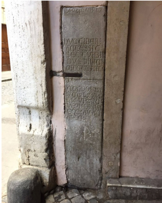
Fig. 24 - The marble slab at Arco dei Banchi: the horizontal line marks the water level of the 1277 flooding. Note in the upper part a posthumous inscription dated 1640.
