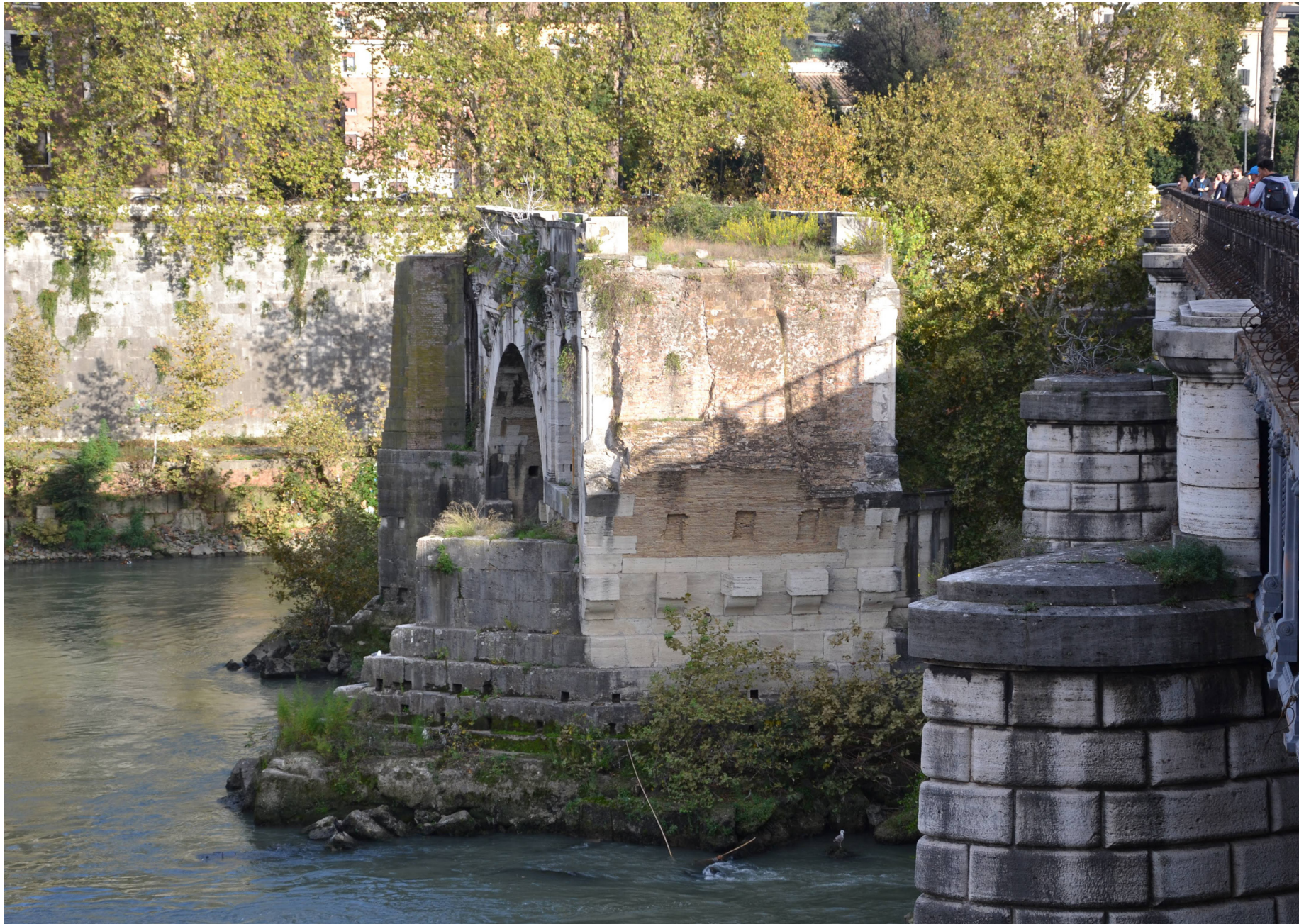
Figure 37 - The remains of the Ponte Emilio, now commonly known as “Broken Bridge”, destroyed by the flood on Christmas Eve of 1598.
