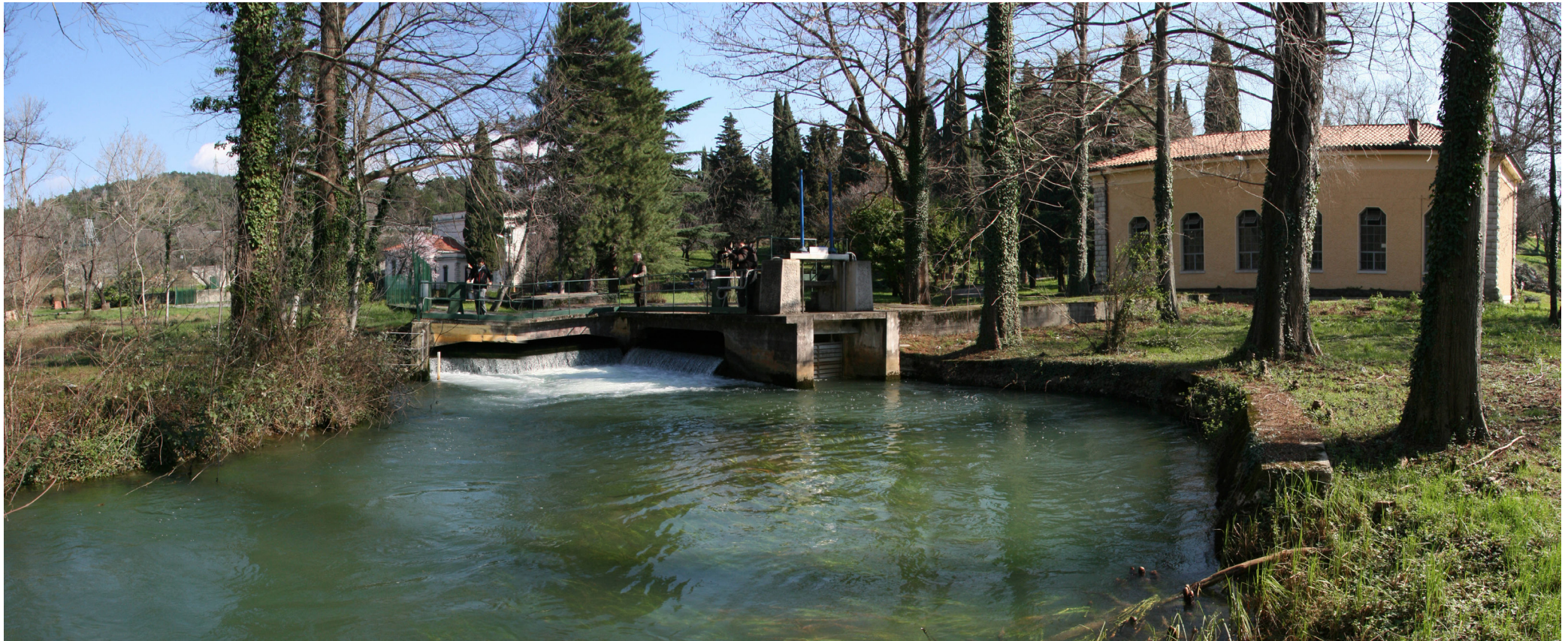
Fig. 41 - Sardos springs: the outflow inside the Randaccio water supply plant.
