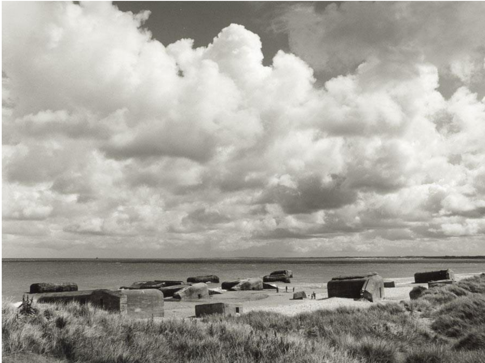
Fig. 12 - A view from land towards the sea at Vigsø in 1970. The location of the World War2 bunkers was used to estimate the coastal retreat to approx 3 \text{ m y}^{-1} . People on the beach for scale.
