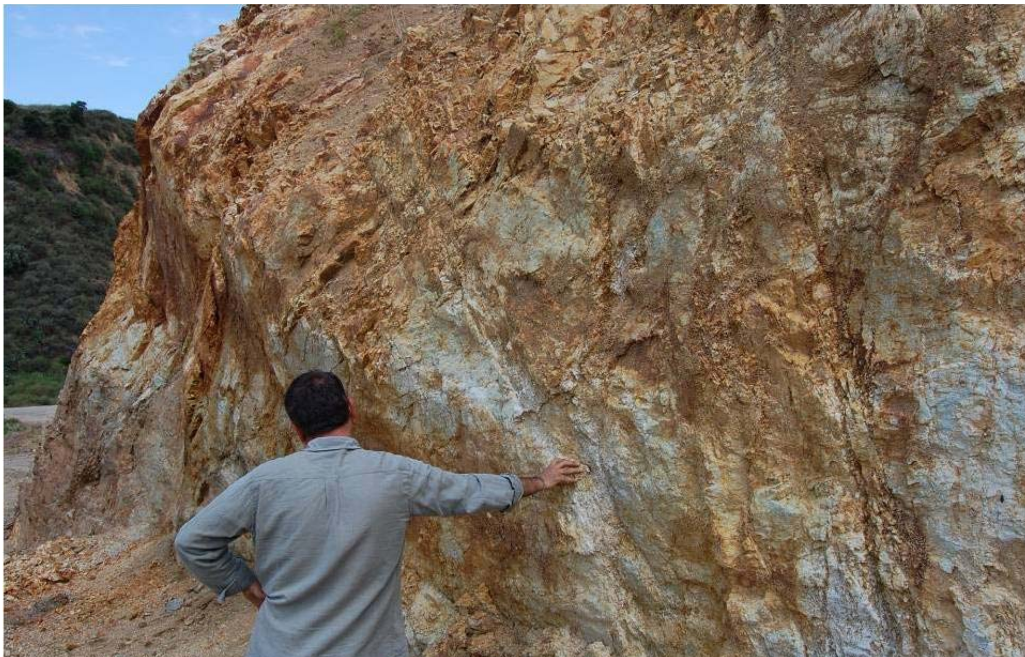
Fig. 23 – NW-trending left lateral strike-slip fault in the metamorphic substrate of the Arente River area (Crati Valley).
